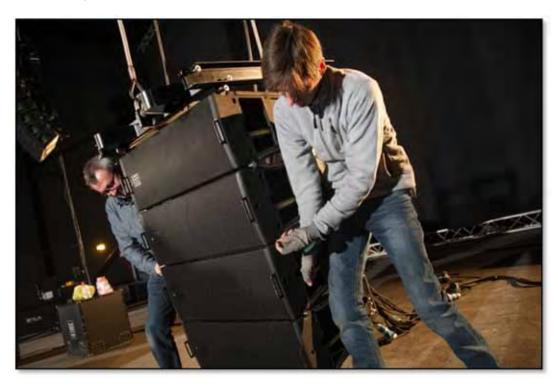
Remove the wheelboard then connect power to cabinets 2 and 3 but NOT 4, as we have mentioned, the Ceeform on the lower cabinet will make it difficult to rig the next pair of Compact. Connect link cables from cabinet 2 to 3 and 3 to 4, check that they power up correctly and that you get U-Net LEDs illuminating on all powered cabinets.
