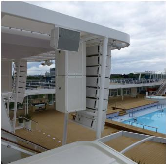
This space required three separate, switchable sound systems: a main Left/Right O-Line hang, with subwoofer support for band set-up; an additional cinema surround, for when the room reverts to movie mode and an acoustic control system to set the venue for different reverberation times — for instance when a string quartet or piano soloist are performing.
