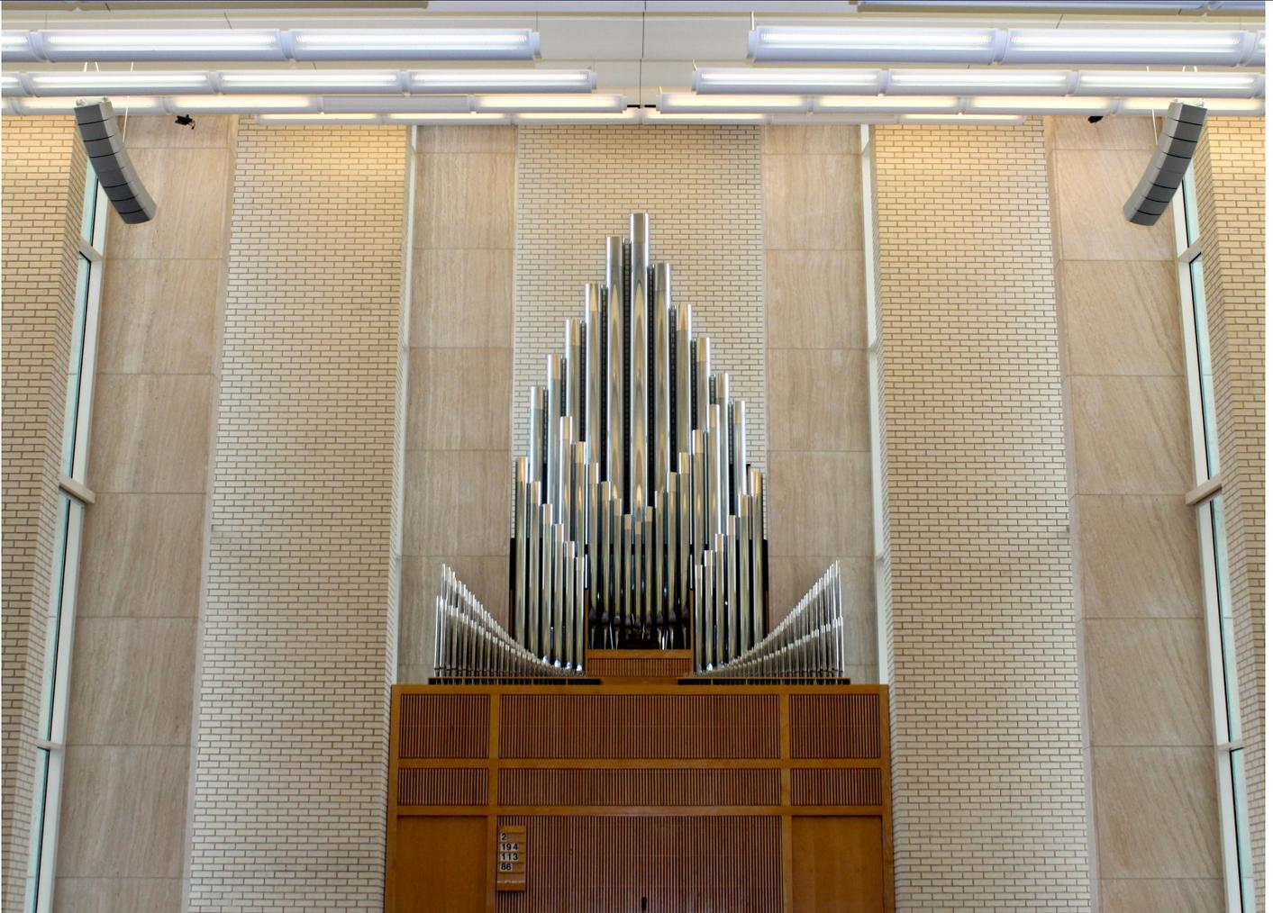
850. Two discrete eight-module O-Line hangs on either side of the rostrum cover the chapel along with two AQ210 subs under the stage.
